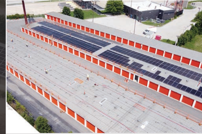
Self Storage: 4MW
