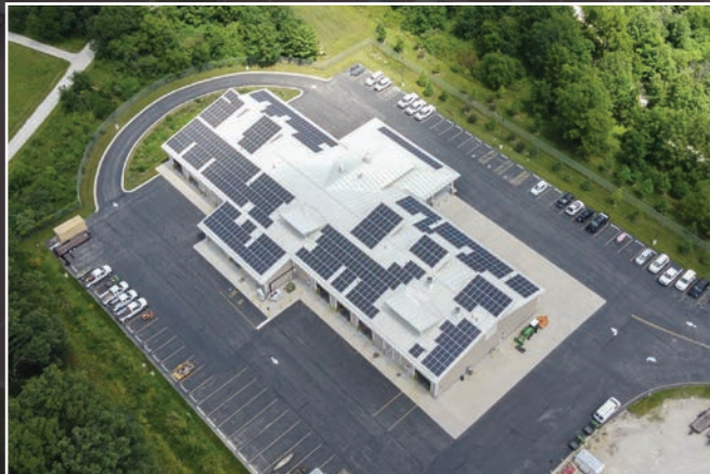
Public Works: 260KW
